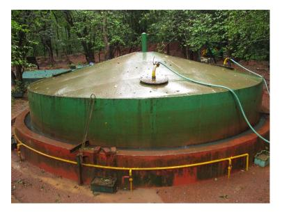
Figure 22. Floating Drum Digester
