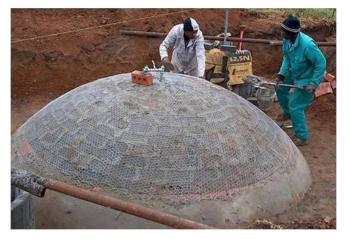
Figure 18. Fixed Dome Digester During Construction Source: Mantopi Lebofa, 2006.
